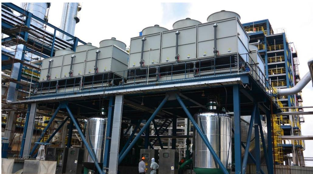
**Fig. 4:** the hot medium water ORC power plant installed at Sinopec Hainan Refinery, Hainan Island, China
